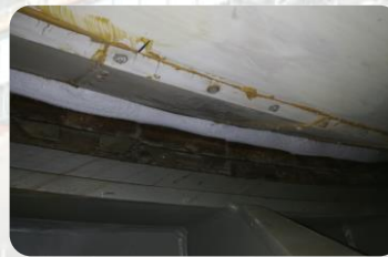
Moisture & Ice Accumulated by Low Temperature
